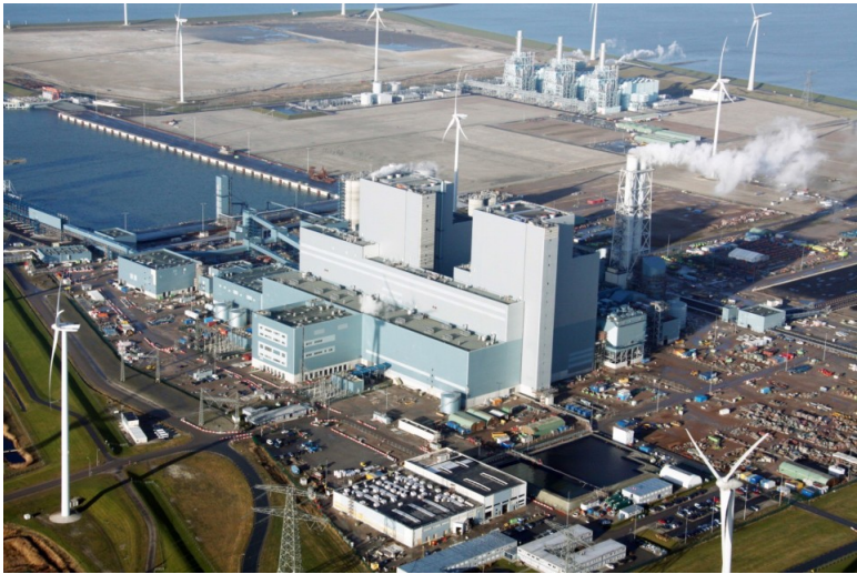
Figure 3: Eemshaven: 2 by 800 MW USC coal plant, 46.2% efficiency
