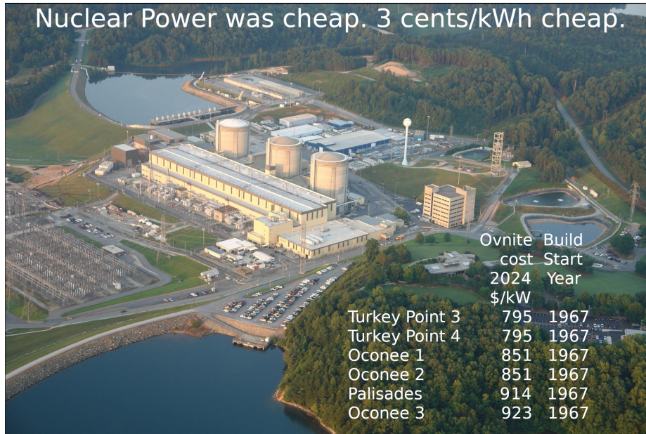
Figure 1: The 2.5 gigawatt Oconee plant in South Carolina. These three reactors were built for just over 350 million dollars between 1967 and 1974. That’s $1141 per kilowatt in 2024 dollars. They took about 6 years to build. Oconee can produce reliable, on-demand, zero pollution, very low CO2 electricity at less than 3 cents/kWh in today’s money. Oconee’s average capacity factor over the last 5 years was 98.2%. All three of these reactors have been licensed into the 2050’s, a gift from the Greatest Generation. Oconee and its cooling pond Lake Keowee have turned a depressed part of western South Carolina into a second home and tourist magnet.
