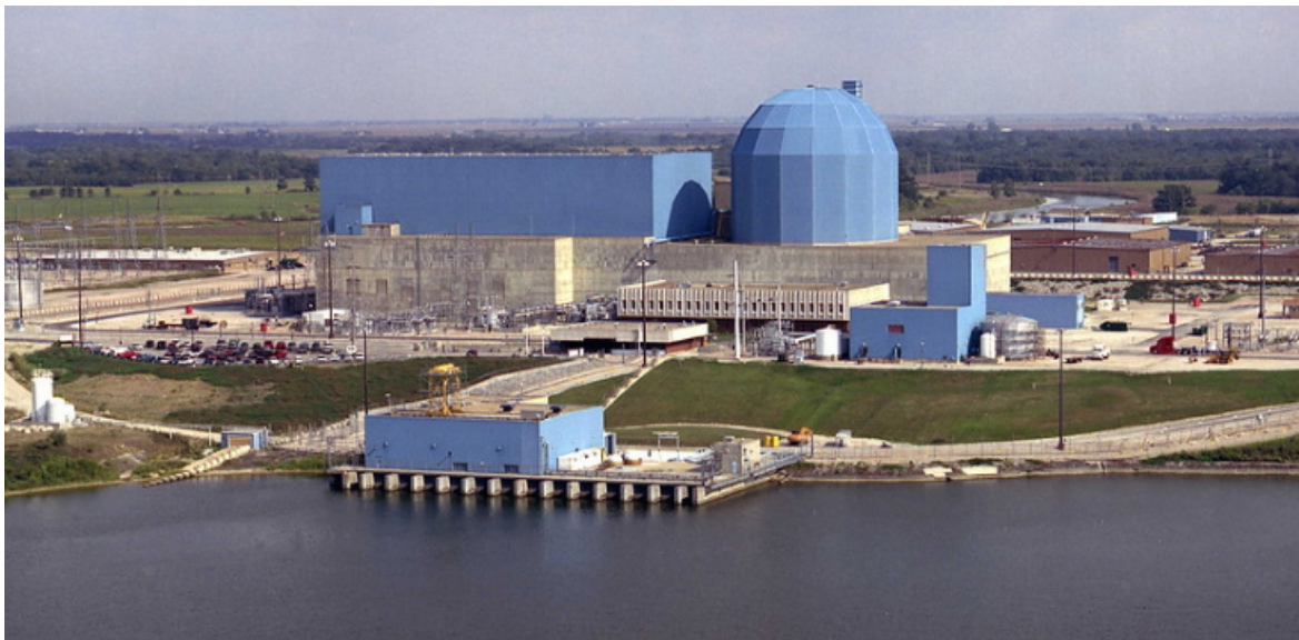
Figure 5: Clinton Power Plant, 1068 MWe, no coal yard, no boiler, no SCR, no baghouse, no big fans, no scrubber, no big stack. Clinton sits on a 5000 acre artificial lake, which serves as its cooling pond. The lake is surrounded by trails, beaches, and a wildlife preserve. It supports active rowing, fishing, and sailing communities. Every fall the lake hosts the Glow Regatta, which attracts sailors from all over the Midwest. Glow is short for Glow-in-the-dark, a cheeky thank you to the lake's mother.
