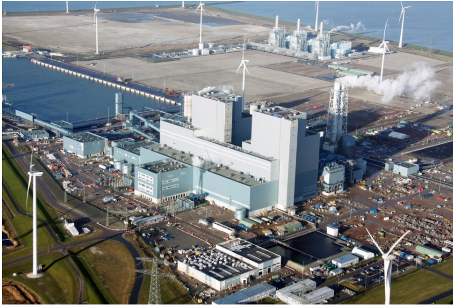
Figure 9.15: Eemshaven: 2 by 800 MW USC coal plant, 46.2% efficiency
