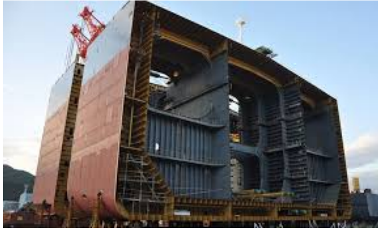
Figure 10.2: Two super blocks in building dock
