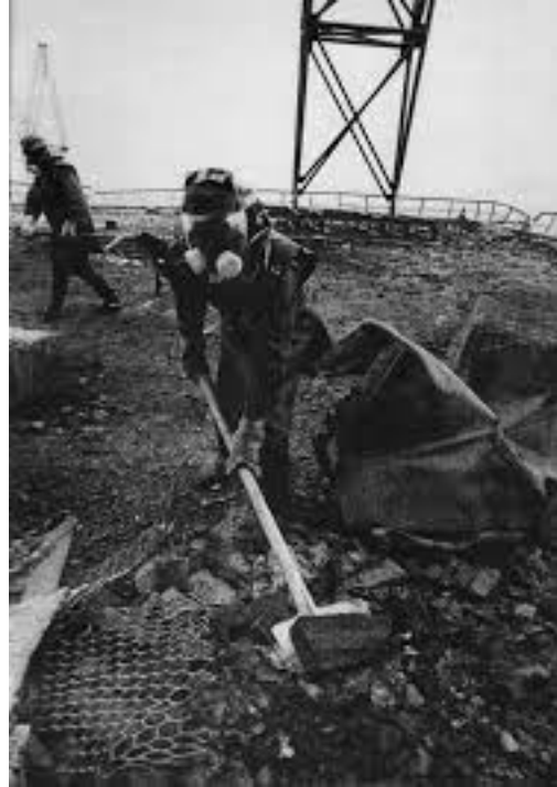
Figure 5.18: Liquidators on Unit 3 Roof
